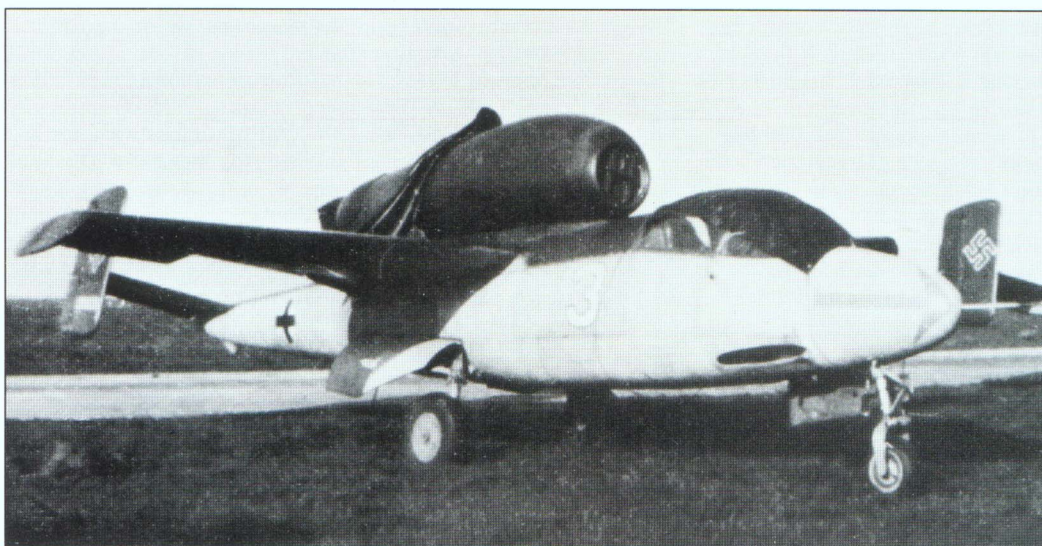
He 162A-2 “White 3” Werk Nr. 120028, wearing the older style of fuselage cross. The upper surface camouflage colour was painted from the cockpit level, aft. Leck 1945
